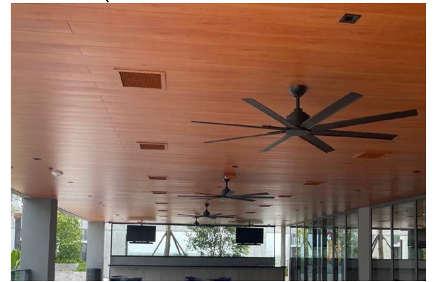
Conditioned Supply Air & Exterior Fans* *Power and Plenum provided by LL Fans, HVAC units and distribution furnished and installed by Tenant
